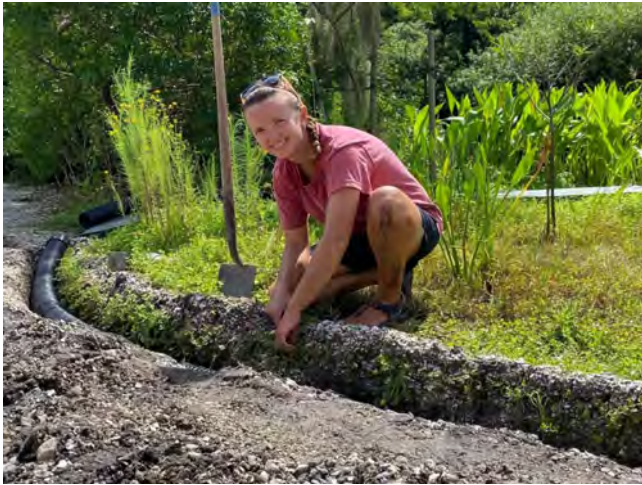
SCCF Installing drainage for the garden.
